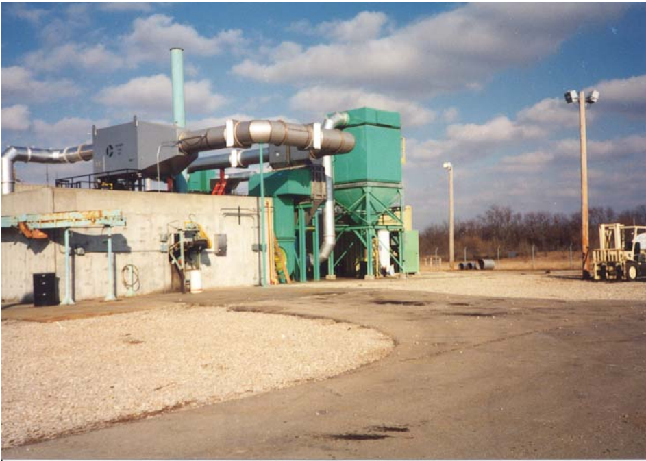
Waste Gas Afterburner & Heat Exchanger installation At Hawthorne Army Depot, Nevada
